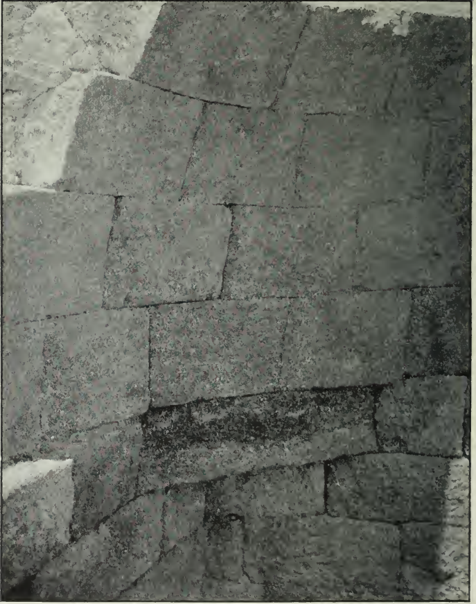
FIG. 205.—Mahaletch, setting of dome.
